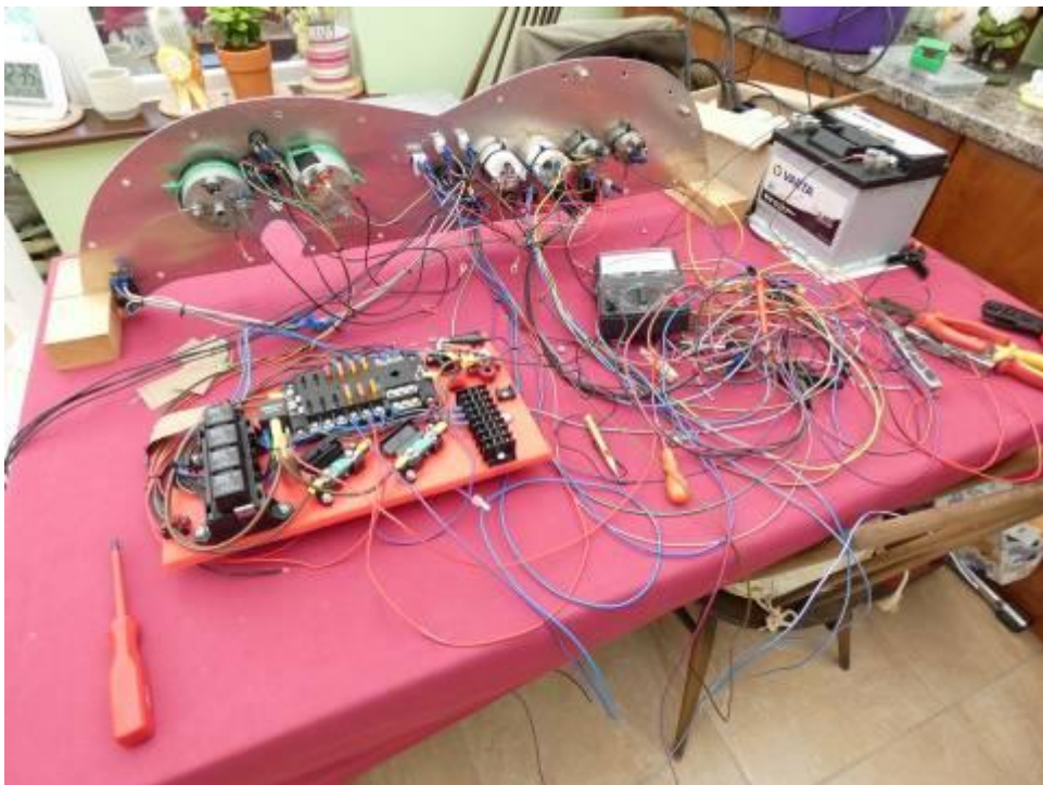
The wiring looks a bit of a mess.
