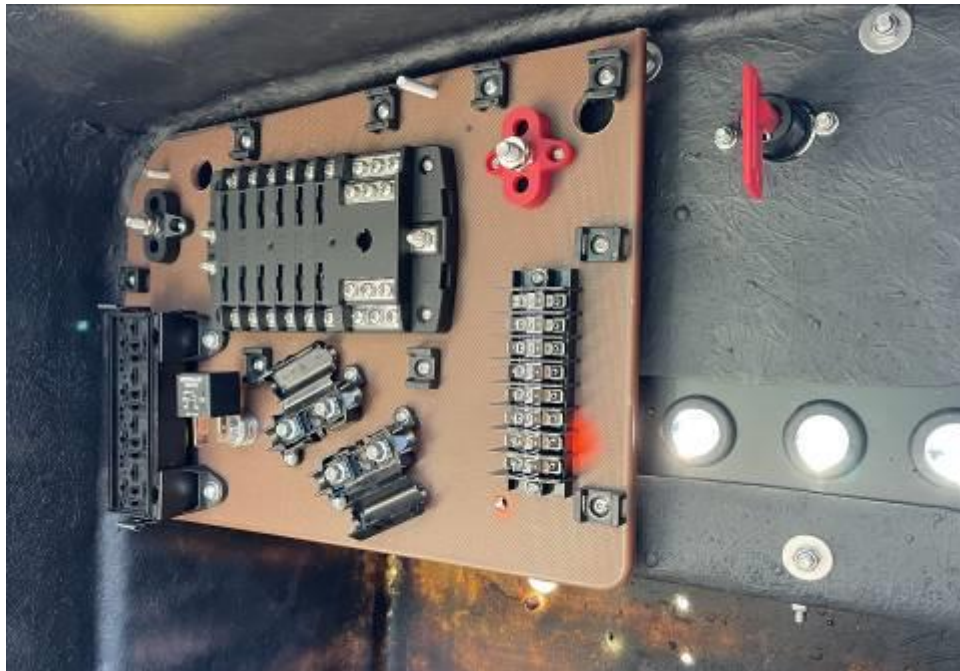
Trial fitted in position.
